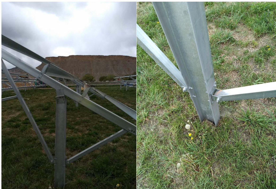
Figure 6. Solar PV racking with a single support pile.
