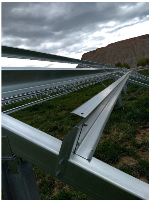
Figure 9. Cold rolled steel support structures are lightweight but can be weak along certain axes.
