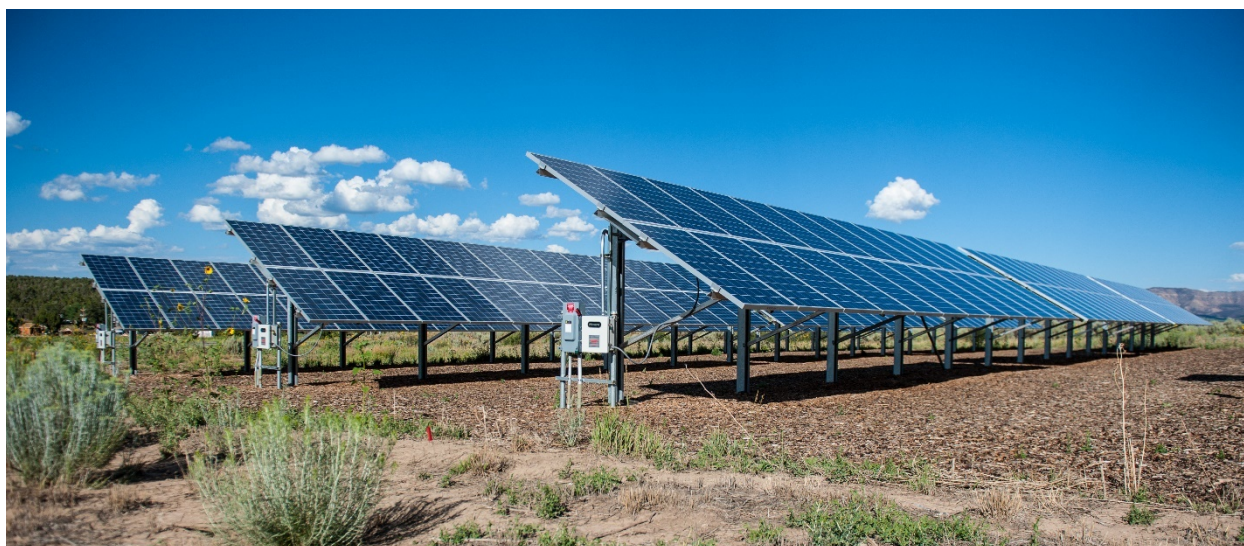
Figure 7. A ground-mount solar array using a dual pier support system
