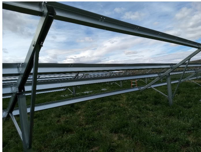
Figure 5. Standard two-rail racking frame
